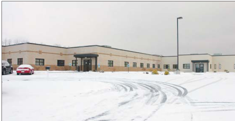
DAVE PRELOSKY/BUTLER EAGLE Western PA Child Care in Allegheny Township, a youth residential treatment facility, is planning an expansion of 24 beds this spring, raising the number of students that can be housed at the facility to 96. The center has a secure area stay program for youth that are flight risks, as well as a shelter program for those awaiting court-assigned locations for treatment. The facility has a waiting list of about 30.
